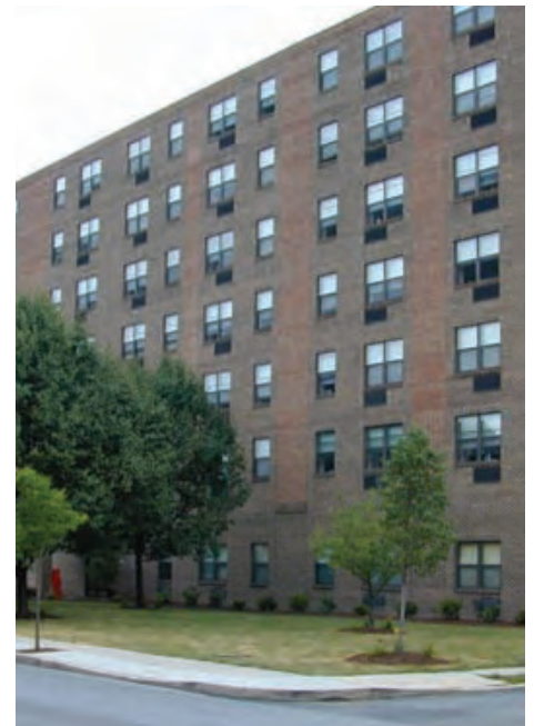
Laurel Towers provides affordable housing for the elderly in Harrisburg.
